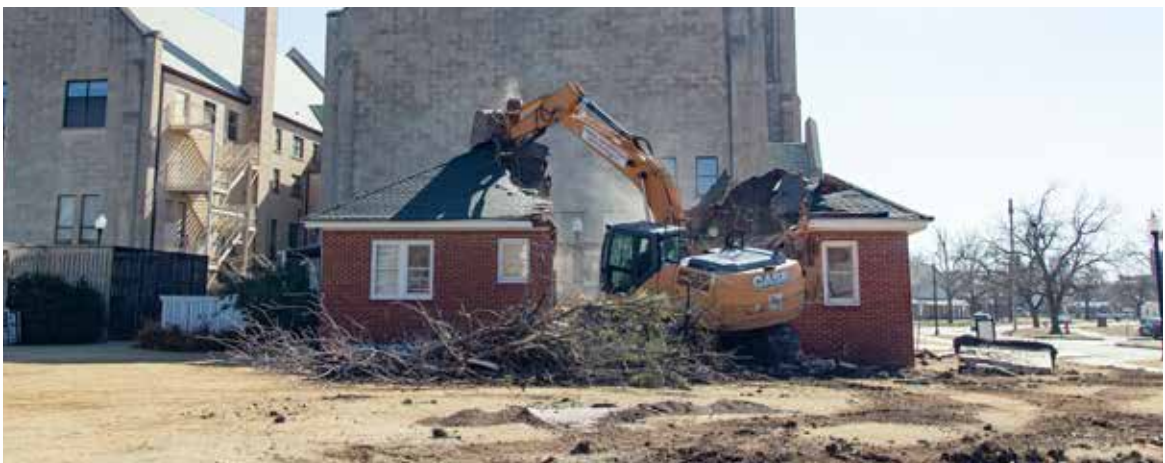
Demolition of The Aldersgate House 2023
