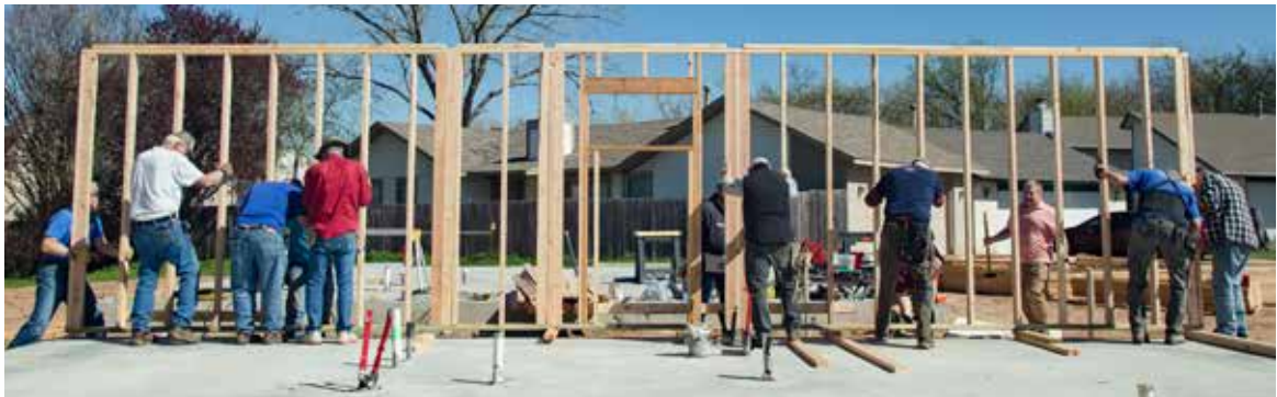
Building of the Habitat House 2023
