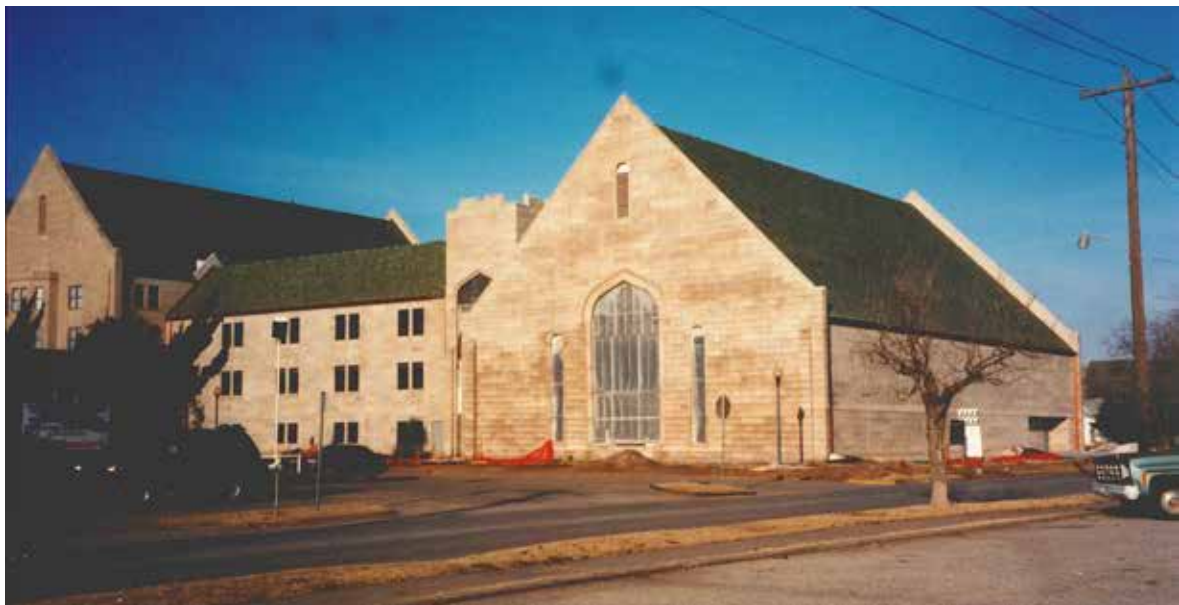
New Building Construction 1999-2000
