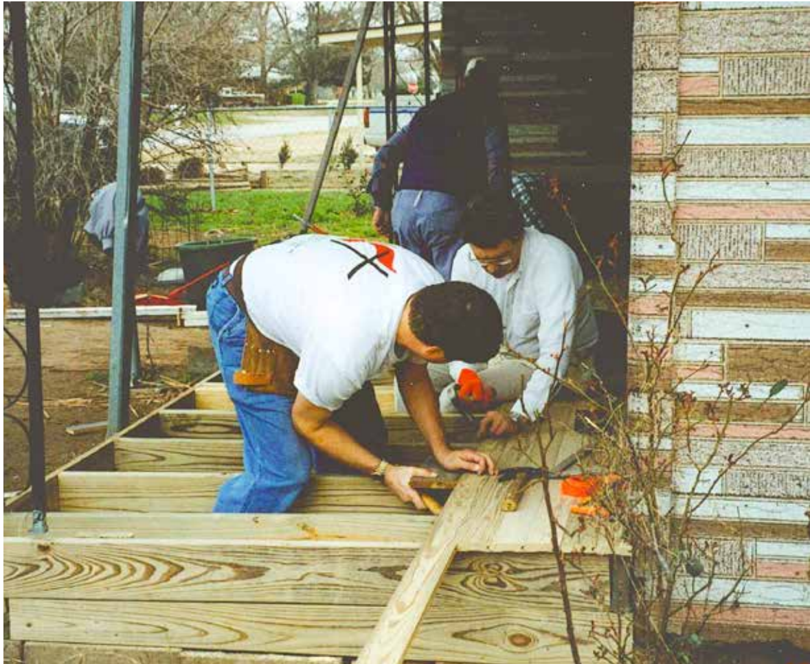
UMM Building a Ramp 1998
